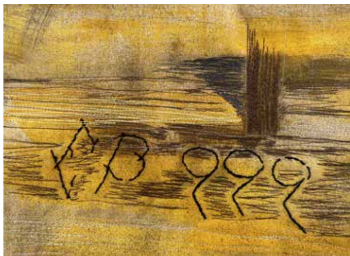
Left: Carpenter's Marks
